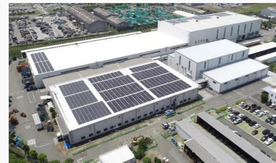
< Front > Logistics building < Back > Plant building
